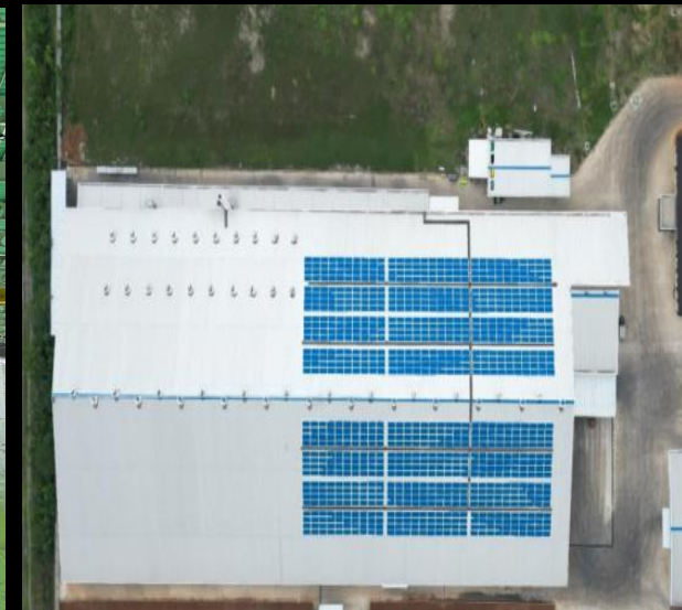
Solar Power Generation Facilities
